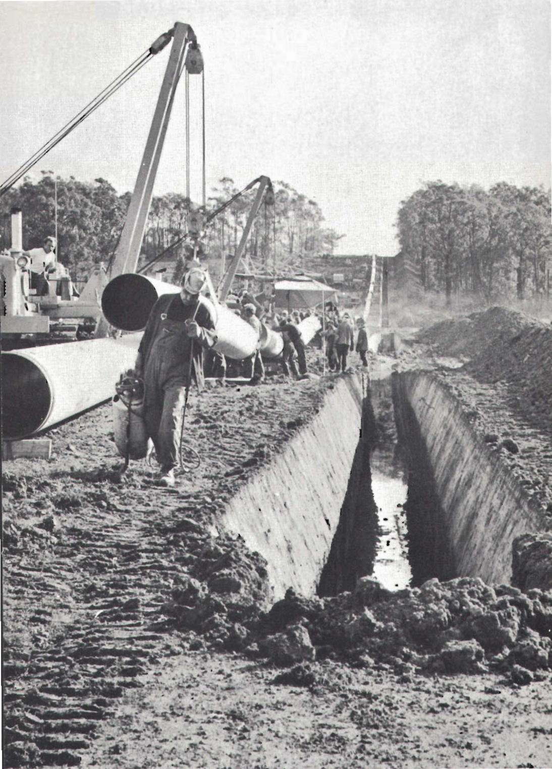
Laying the natural gas pipeline from Gippsland to Melbourne.
