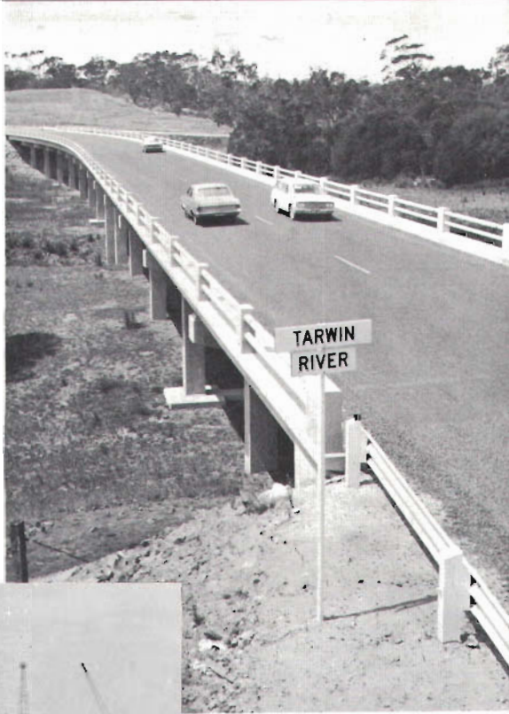
New concrete bridge on the South Gippsland Highway over the Tarwin River near Meenyan. [Country Roads Board]
